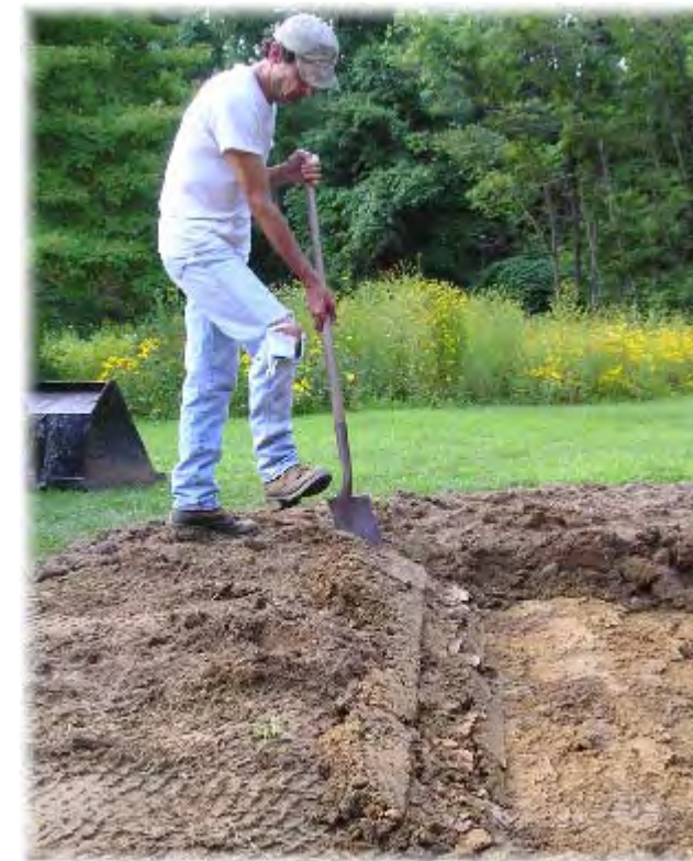
You can dig your rain garden by hand or use a backhoe. If you use a backhoe to dig your garden, avoid driving it on the garden site to minimize soil compaction.
